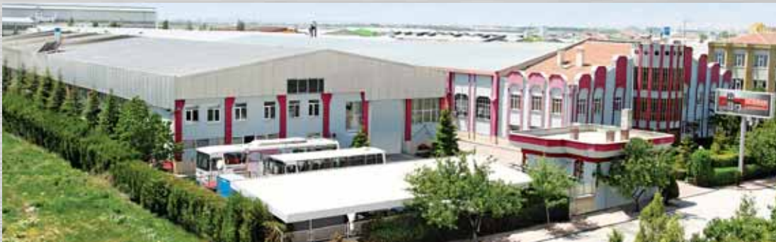
Piston & Piston Pin Production Facility
